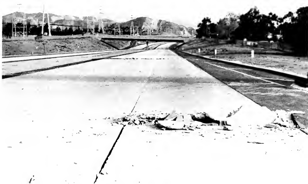
Photo 9. Compression buckles in concrete pavement on Route 210.
